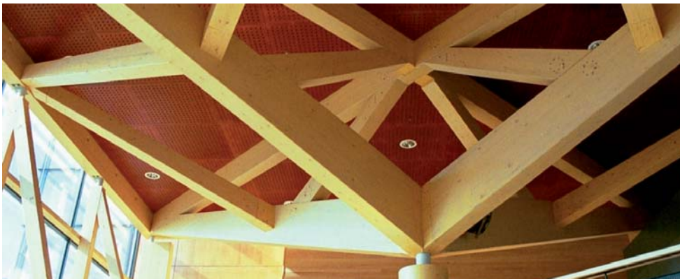
Designing timber roof structures such as this to Eurocode 5 should be simpler and safer with the forthcoming TRADA / IStructE design manual
