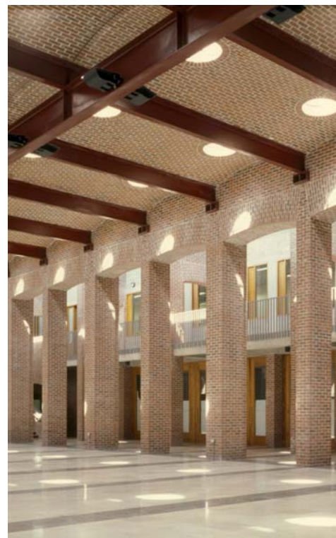
Eurocode 6 and support resources produced by the industry is likely to encourage greater use of structural brickwork, such as the recent award-winning Cork Institute of Technology
