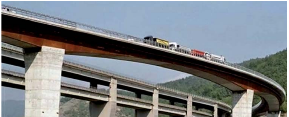
Completed in 2006, the Roccaprebalza viaduct on the A15 motorway in Italy was designed to EN 1992-1-1, EN 1992-2, EN 1994-1 and EN 1994-2.
